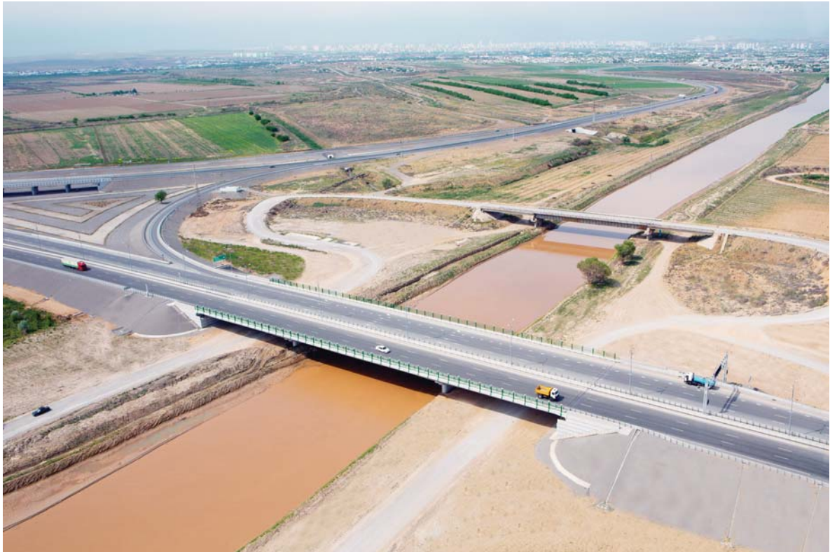
Bridge across the Karakum River in the alignment of Andaliba street Ashgabat, Turkmenistan
