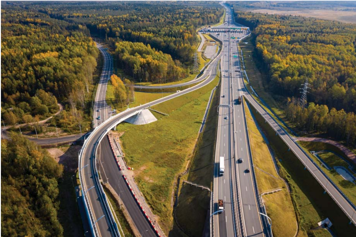
Transport interchange of the Western High-Speed Diameter (WHSD) highway at the intersection with Novoe highway. St. Petersburg
