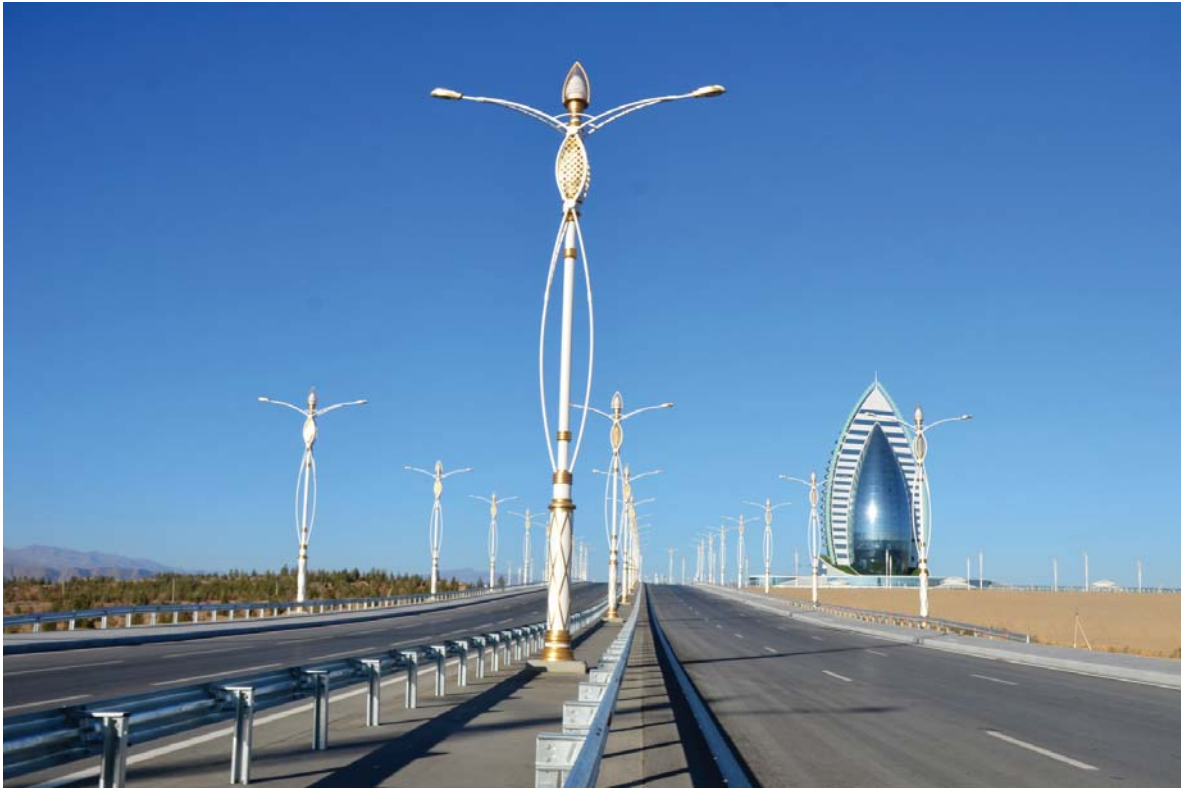
Construction of roads to a five-star hotel Ashgabat. Turkmenistan
