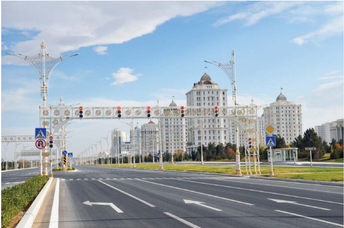
Reconstruction of Archabil Avenue Ashgabat. Turkmenistan
