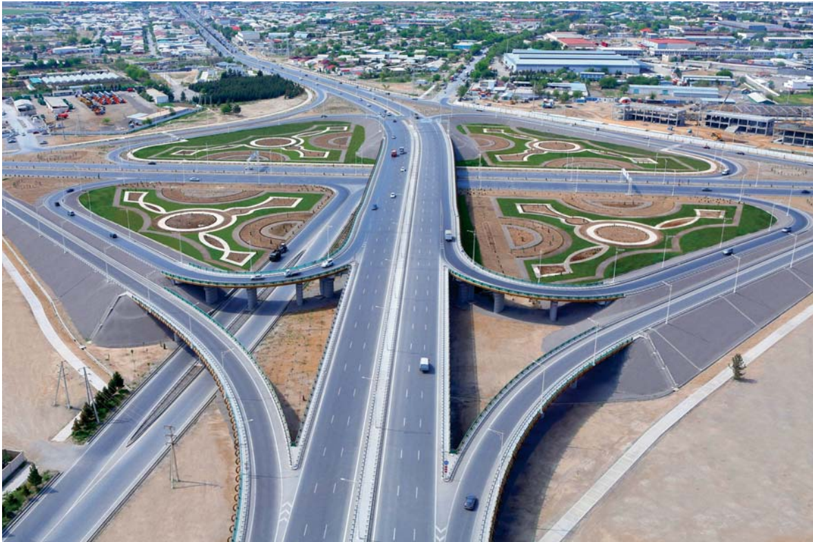
East-West Transport Corridor Ashgabat, Turkmenistan
